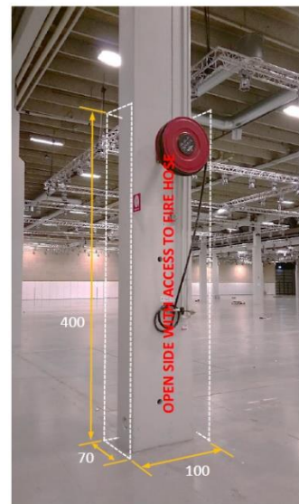
SELF-STANDING BOX TO COVER PILLAR ON 3 SIDES NEXT TO ARCADE C3/C4
