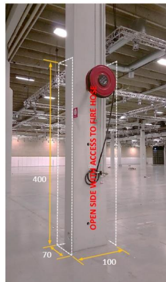
SELF-STANDING BOX TO COVER PILLAR ON 3 SIDES NEXT TO ARCADE C3/C4
